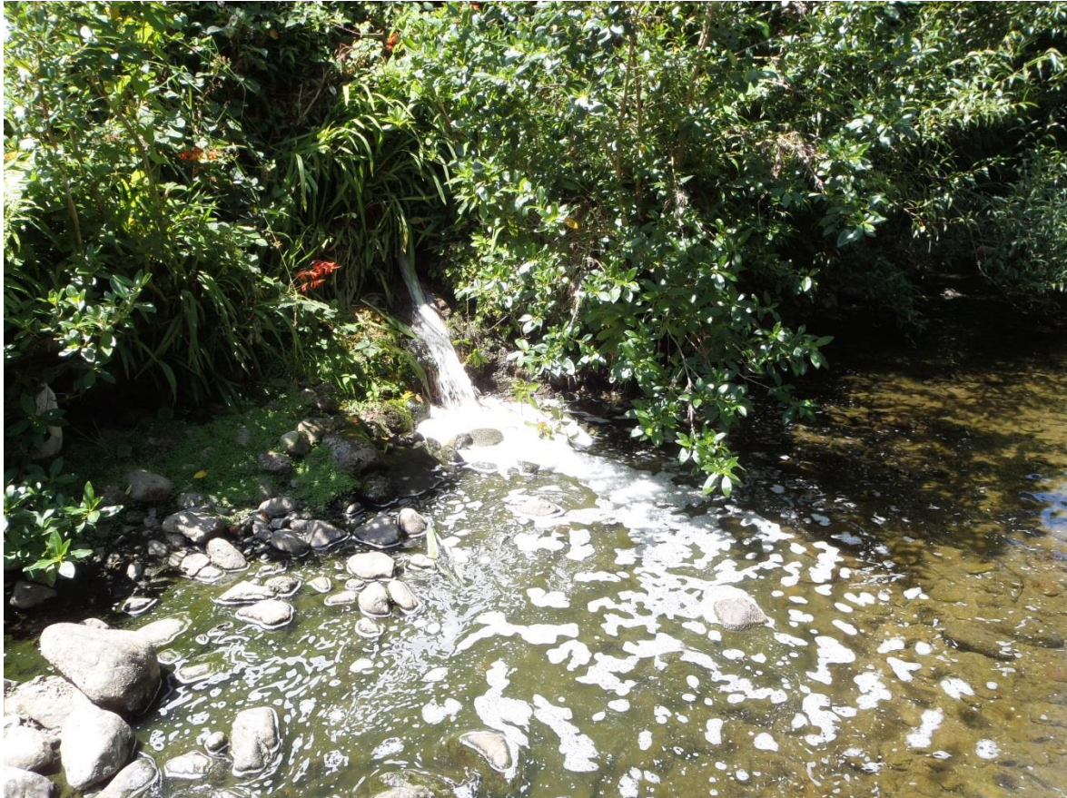
Photo 1: Current discharge structure from the Eketahuna WWTTP into the Makakahi River.
